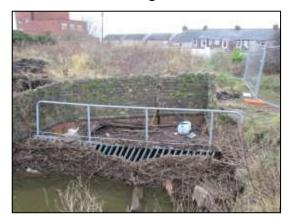
Figure 22: Risehow Beck grid - erosion on left bank Figure 23: Risehow Beck grid - erosion on left bank
