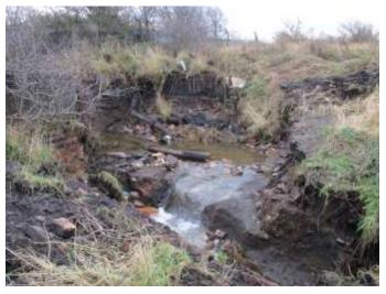
Figure 24: Erosion behind Risehow Beck grid
