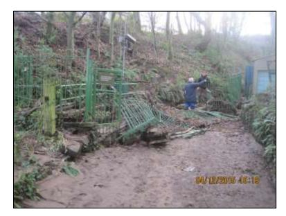
Figure 10: 6 Allanby Close culvert blockage
