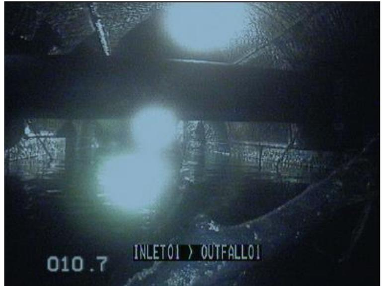
**Figure 6. Picture from CCTV survey showing service pipe passing through the culvert and a branch caught on it**
