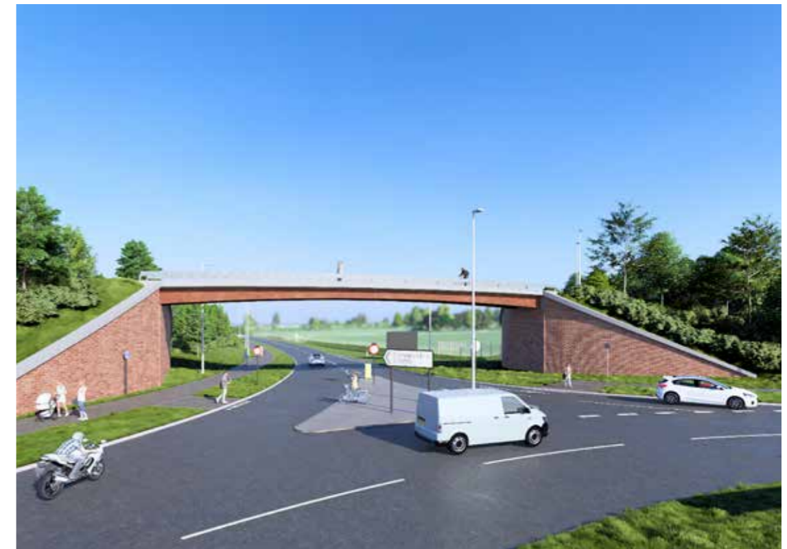
Curved sandstone wing walls and corten steel cross beams on Dalston Road
