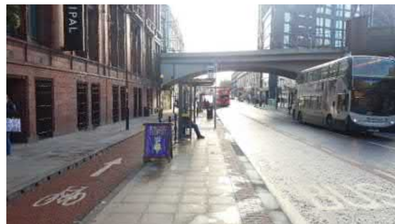
Figure 3.7. Segregated cycleway (carriageway height)
