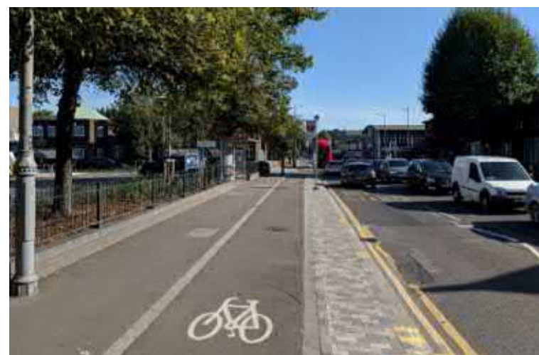
Figure 3.8. Stepped cycle track (intermediate height)
