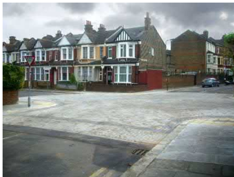
Figure 4.9. Raised table junction
