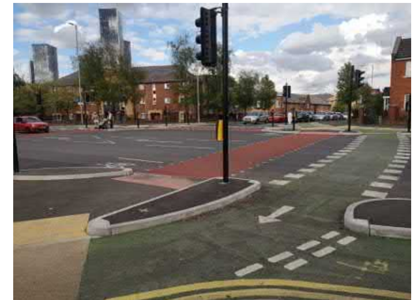
Figure 3.13. CYCLOPS signalised junction
