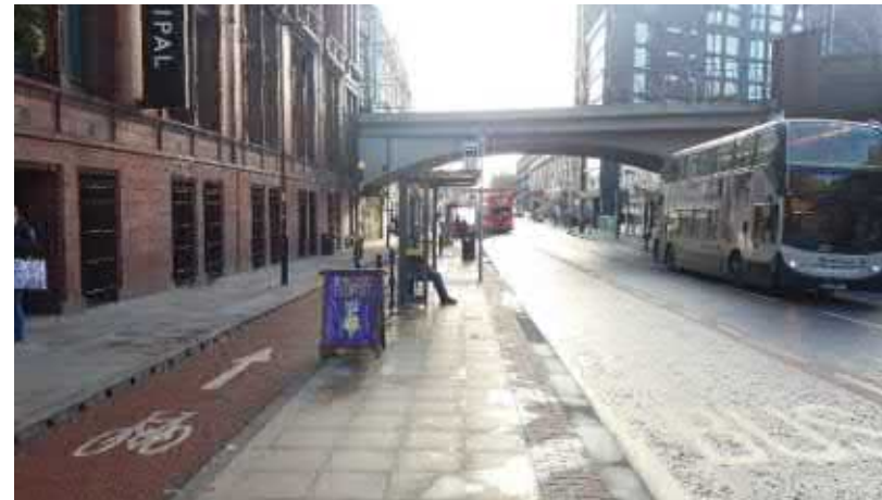
Figure 3.8. Segregated cycleway (carriageway height)
