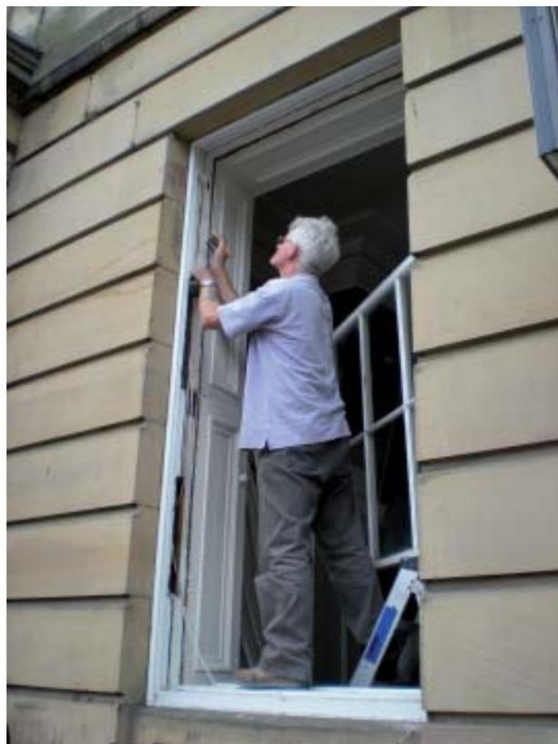
▲A sash window is designed to be easily removed for painting/maintenance.
